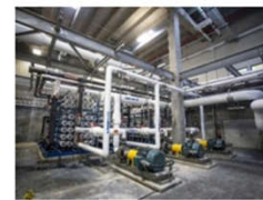
Figure 5.3.3: Typical High Pressure Membrane System
